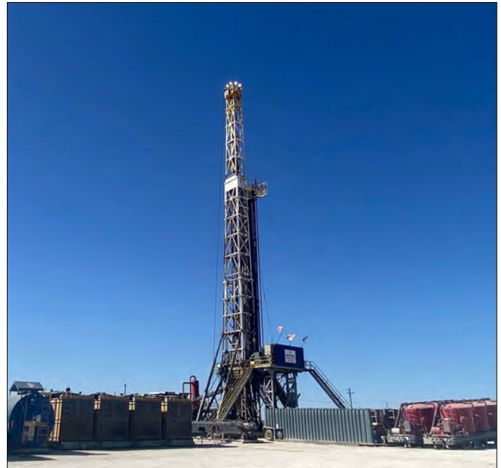
Becky 1H Drilling Location - Pradera Fuego Project Permian Basin, Ector County
