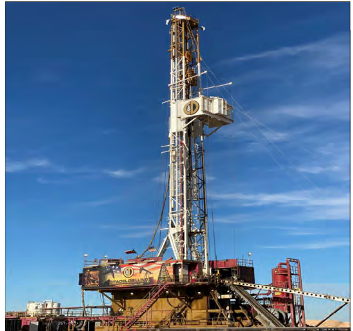
Ava Unit 1H Drilling Location - Pradera Fuego Project Permian Basin, Ector County
